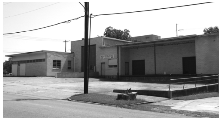
The "before" photo of our new Essential Needs Distribution Center. Currently, work is being done to put this building into operation before the end of November. See more details in the story below.
